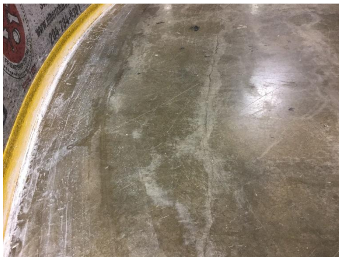
Photo 8: Arena Slab - cracks
