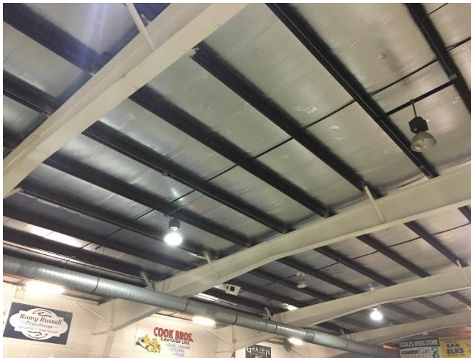
Photo 17: Pre-Engineered Roof Support System – Roof Cross Bracing
