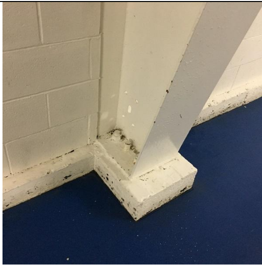
Photo 19: Missing Anchor Bolt Nut
