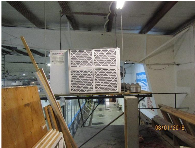
Photo 4: Indoor Dehumidifier Platform
