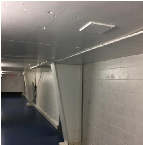
Photo 15: Pre-Engineered Roof/Wall Support System – West Wall Cross-Bracing
