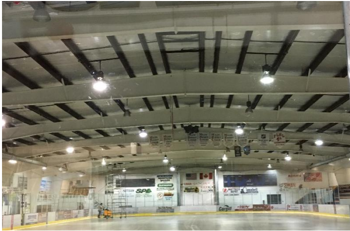
Photo 16: Pre-Engineered Roof Support System – Purlins
