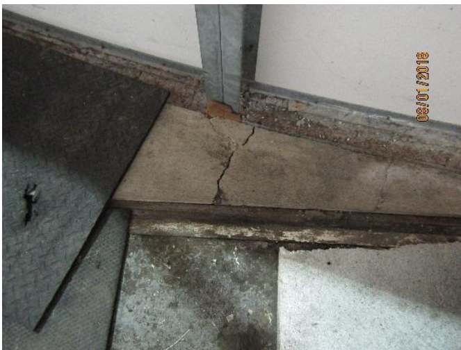
Photo 27: Ring Slab Cracks
