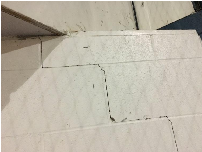
Photo 11: Concrete Block Crack
