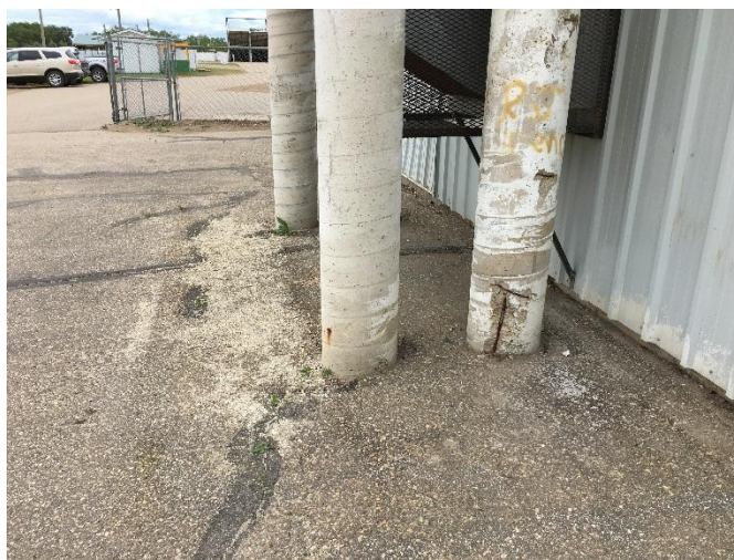
Photo 3: Outdoor Condenser Platform Support Piles
