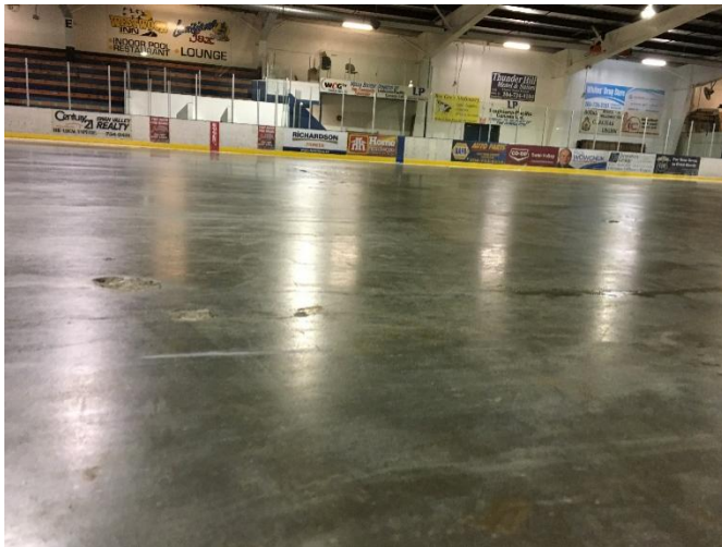
Photo 26: Poor Slab Surface Condition
