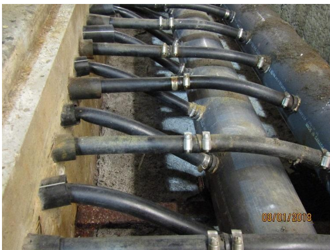
Photo 24: Brine Piping Loops in Header Trench
