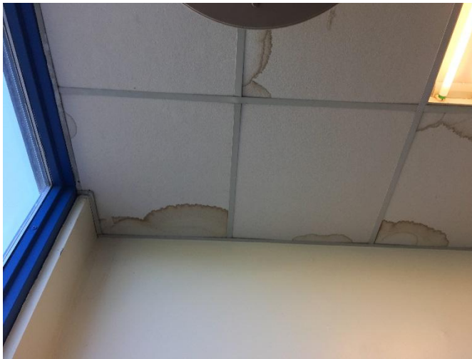
Photo 14: Roof Leak Repairs
