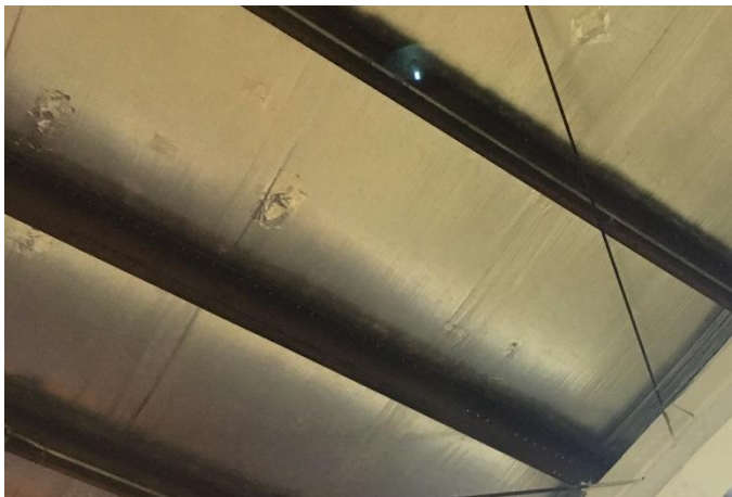
Photo 21: Ceiling Reflective Surface
