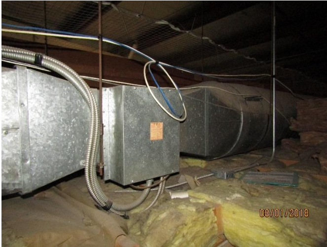
Photo 22: Arena Furnace with re-heat loop
